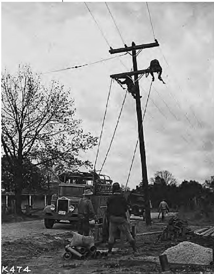
K474 Stringing a rural electricity transmission line during the 1930s.
